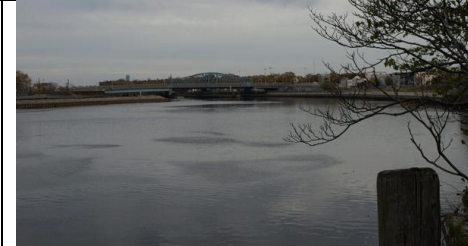
Looking at Jackson St Bridge from upstream
